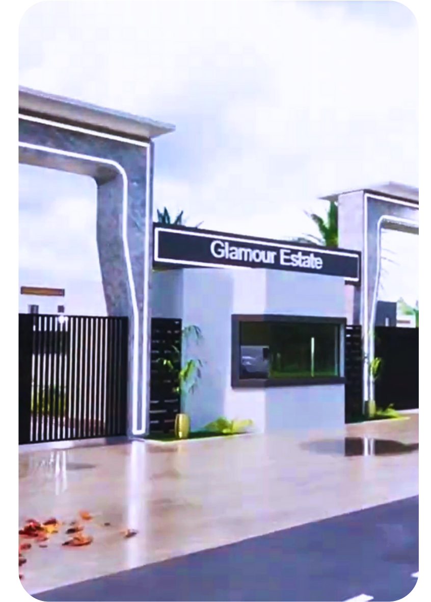
Entrance Estate gate with security checks
